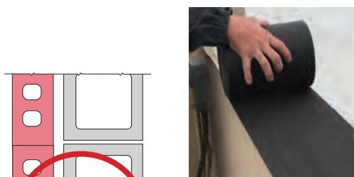
3. Align the membrane's edge with the **exterior** edge of the wall. Cover the entire top of the wall, side-to-side and full length, with membrane. Keep the membrane roll taut as you unroll it 1 to 2 feet at a time. Press membrane into sealant to ensure good bond to wall.
