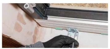
STEP 5: apply a vapor barrier on the inner side of the threshold
